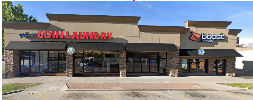
946 S 200 E - Facade Elevation
