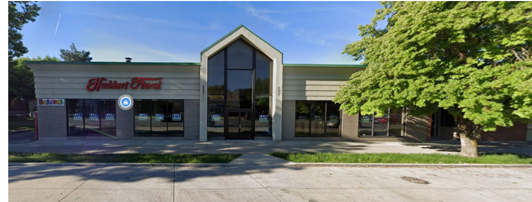
156 E 900 S - Facade Elevation (Project Site)
