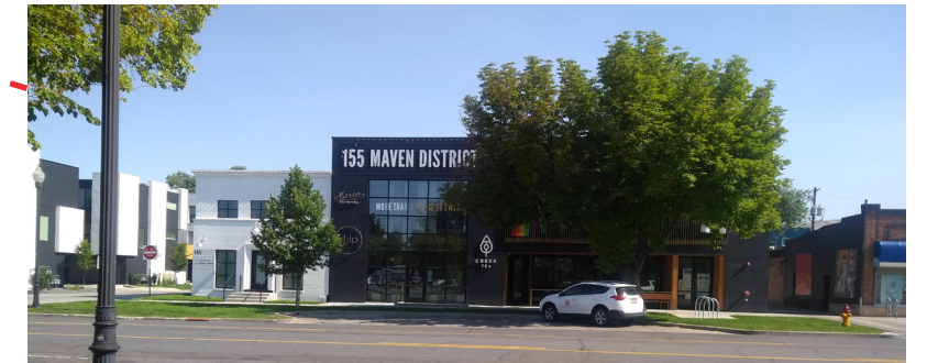
900 S 155 E - Facade Elevation
